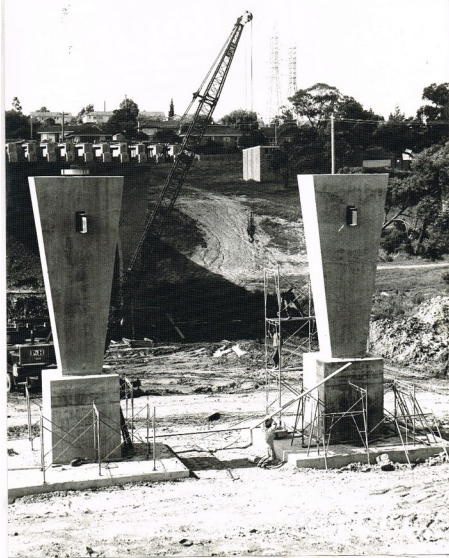
The Stephensons Rd bridge over Scotchmans Creek under construction
